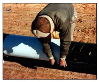
INSULRAP™ 50 Smooth is the premier direct burial membrane in the insulation market used as a waterproofing and vapor-proofing jacketing. Insulrap™ 50 is a "peel and stick" protective membrane. It's made of rubberized asphalt laminated to a white polyethylene film. Using "cigarette wrap" application, Insulrap™ 50 can be shop applied or field applied.
